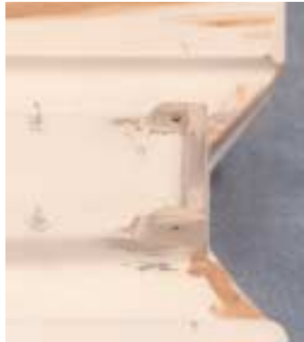
Below: I also used brass inserts and screws to hold the cowl in place. Plywood brackets that I glued to the transom support the threaded inserts.
